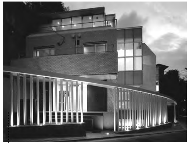
Figure 10. c-MA1, exterior: after (Sources: IKDS)
