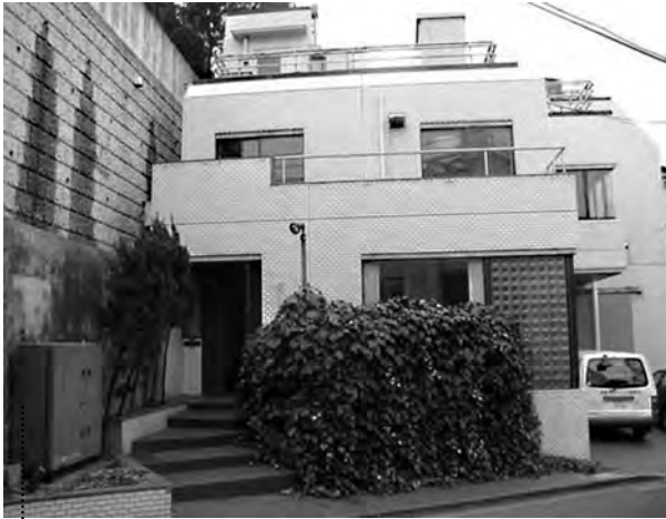
Figure 9. c-MA1, exterior: before (Sources: IKDS)
